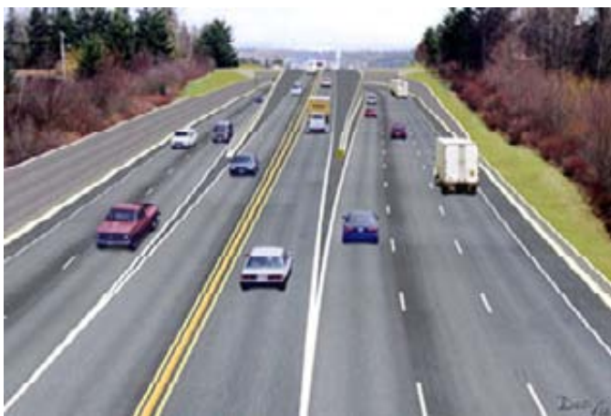
SR 543 as construction is complete.
